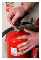
One indicator the fire extinguisher is charged and serviceable is the pressure gauge needle will be located in the green.
